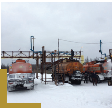
Taymura's oil loading station on site
