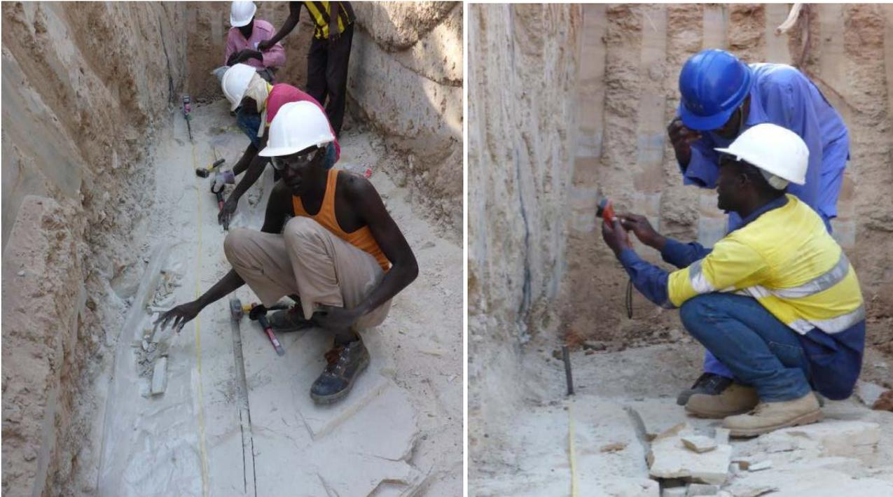
**Figure 4** | Trench sampling underway at Dorothe and training of local Chadian field technicians
