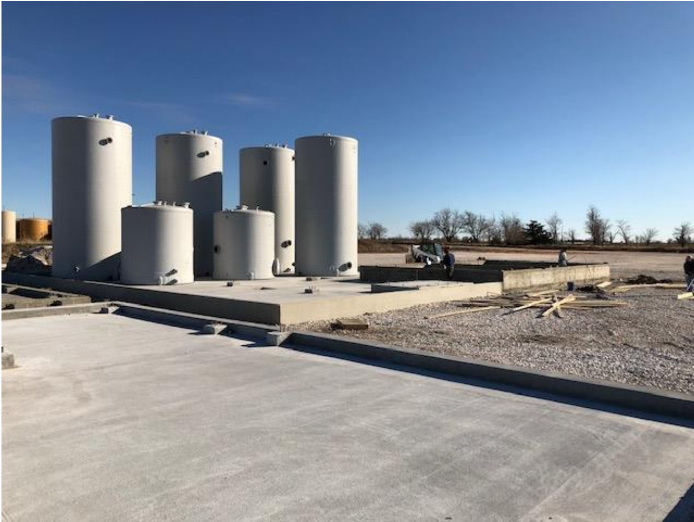
Figure 1. Construction of IO#8 in western Oklahoma
