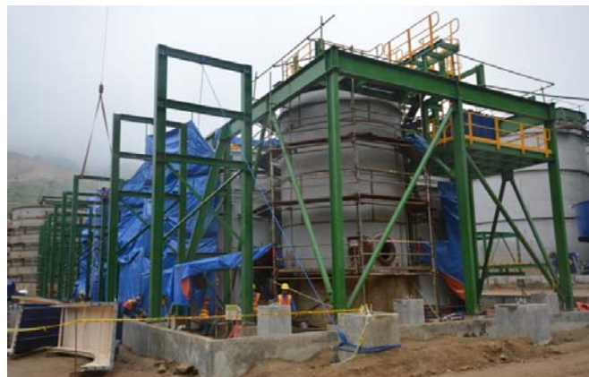
Image 6: CIL tanks and pipe racking
