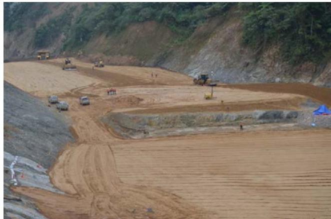
Image11: RSI clay core construction of the dam wall
