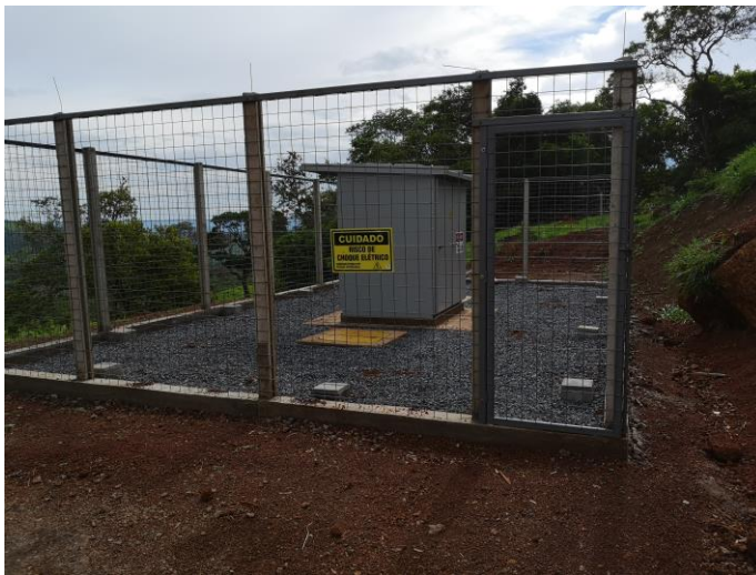
Figure 1: The 600kW substation installed at Arapua and connecting the powerlines.
