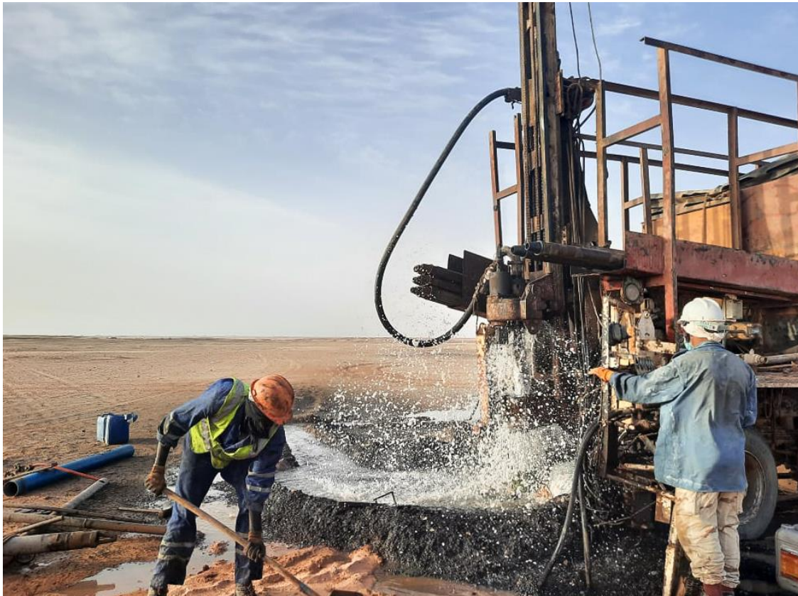
Figure 9 - Water Drilling at the Tiris Uranium Project
