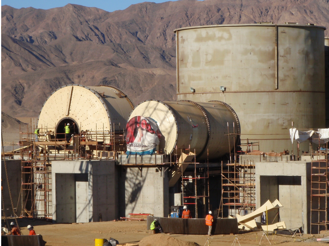
Progress Picture: SAG Mill and Ball Mill 1 in place
