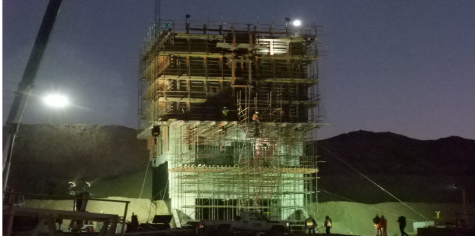
Progress Picture: Primary Crusher civil works nearing completion
