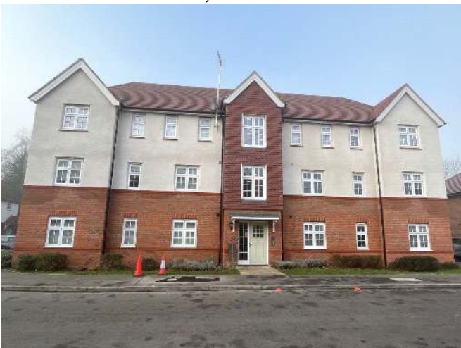
RG2 9UU, Chaucer Grove
