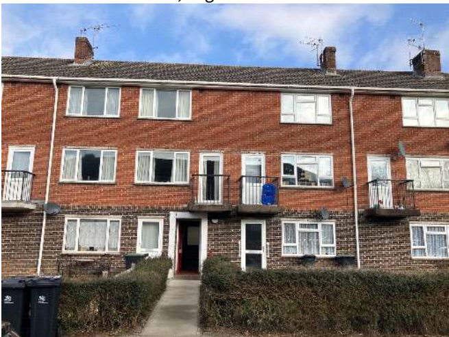
DT11 7BS, Eagle House Gardens
