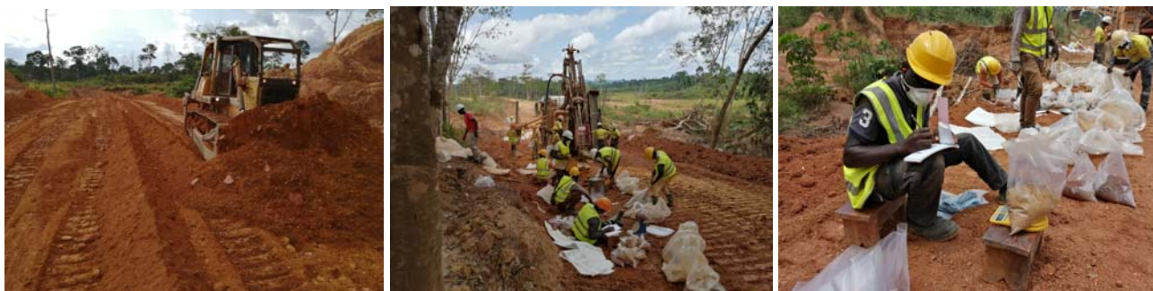
Figure 4: Ongoing access and drill pad preparation (left), ongoing AC drilling (centre) and field logging (right).
