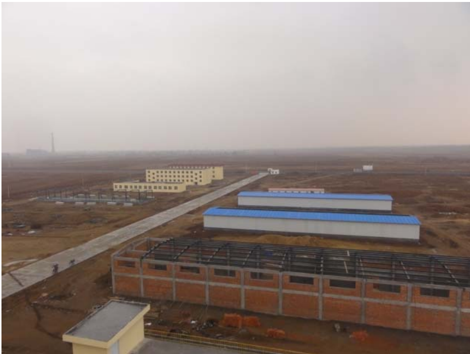
Site of new facility in Inner Mongolia: November 2011
