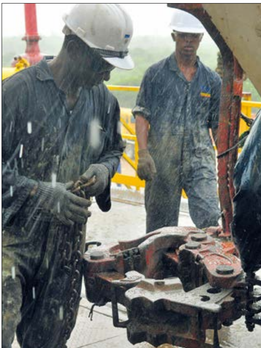
◆ Drilling operations at Ntorya
