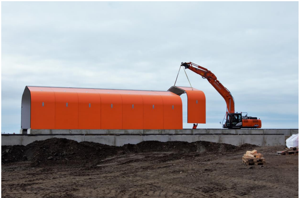
Figure 3: Construction of maintenance and storage buildings
