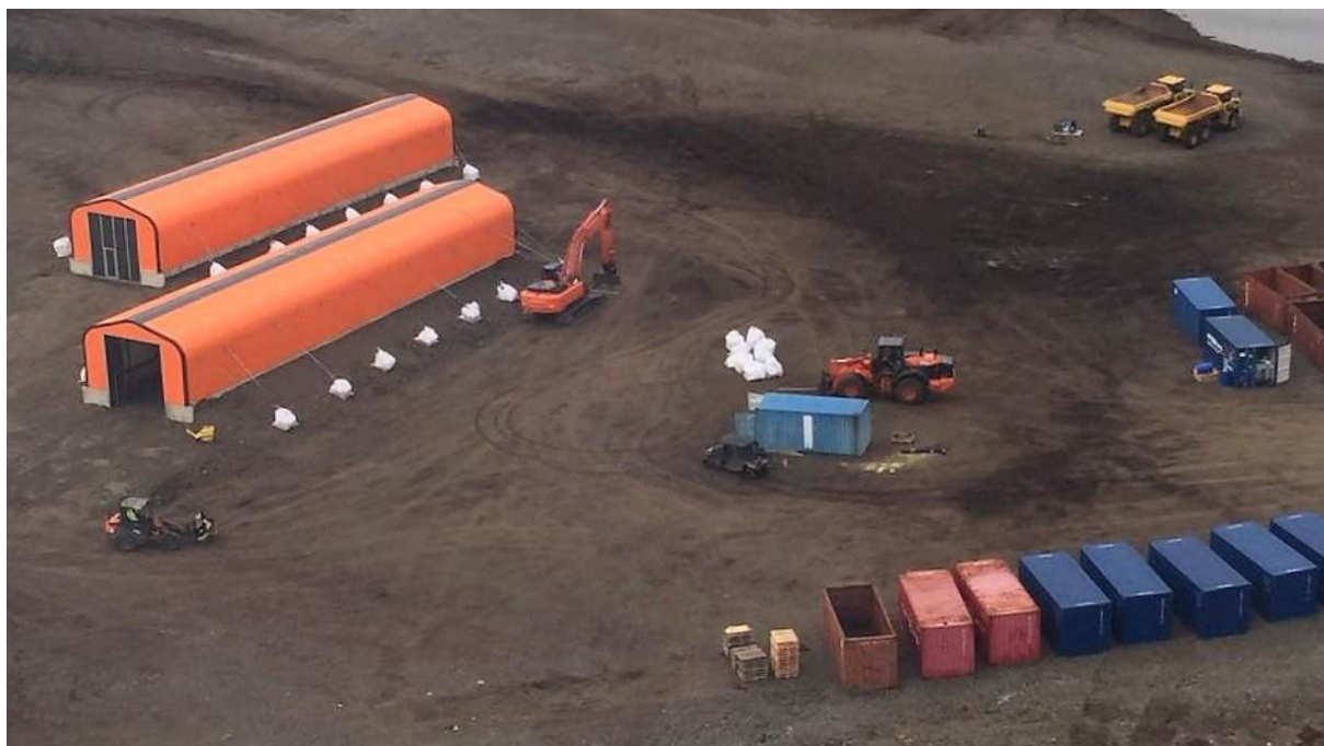
Figure 4: Site work preparation at Dundas
