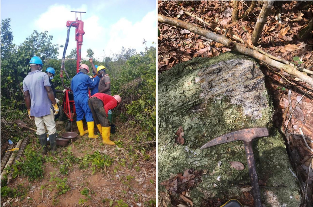
Figure 1: Mechanised auger drill rig active on site (left), example of spodumene bearing pegmatite outcrop observed within a new target area (right).
