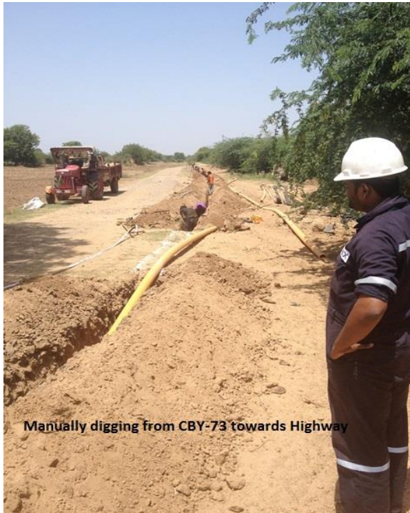
Cambay-73: MDPE pipeline trenching
