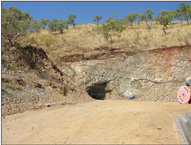
Figure Three | Exploration Portal and Decline Access
