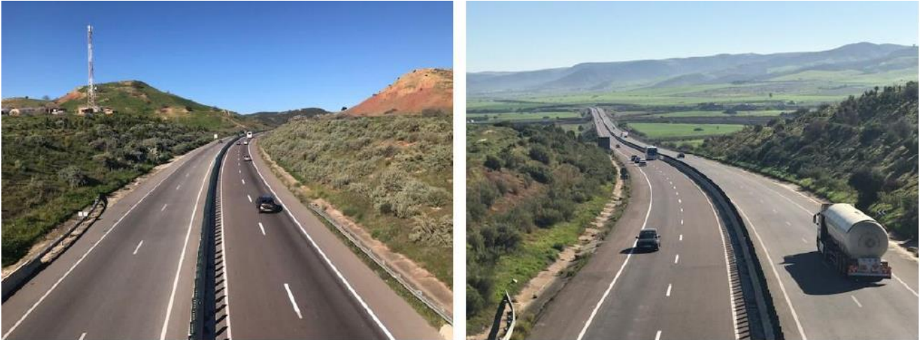
Figure 19: A2 highway road crossing the project area
