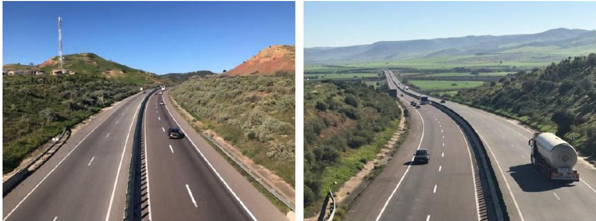
Figure 25: A2 highway road crossing the project area
