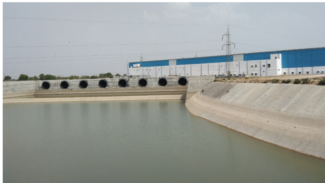
REC funded electro-mechanical and associated civil works at Indirama Flood Flow Canal Scheme in Telangana
