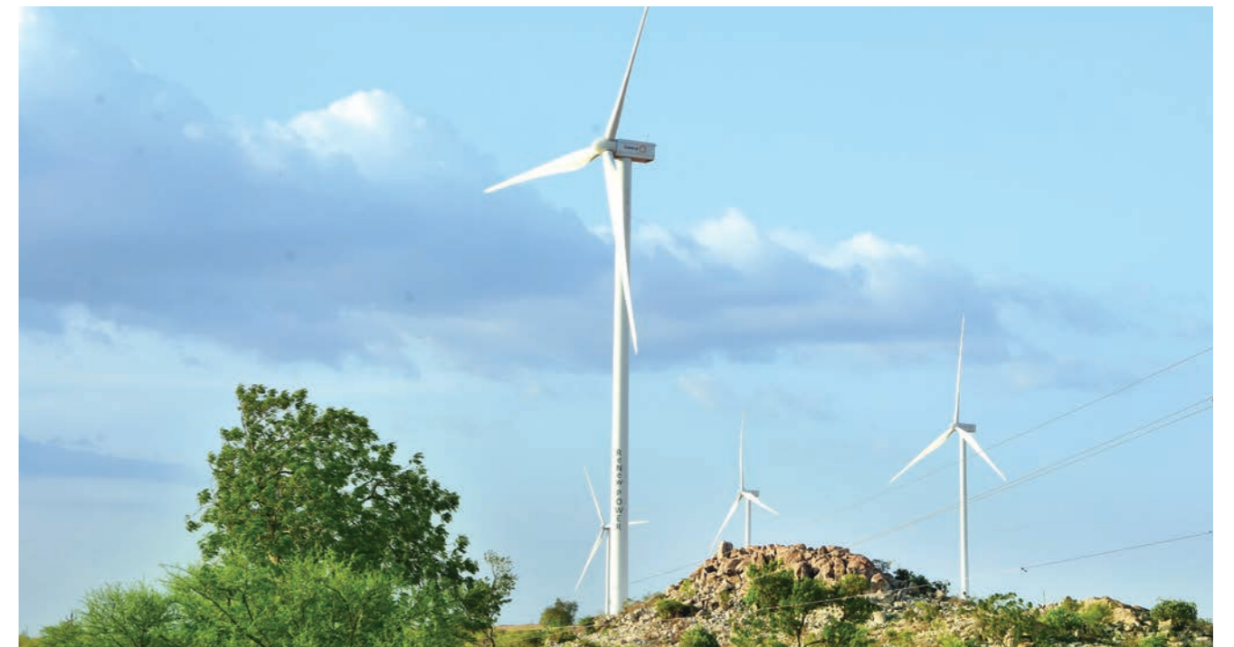
60 MW wind project of Renew Group in Karnataka, which was financed by REC
