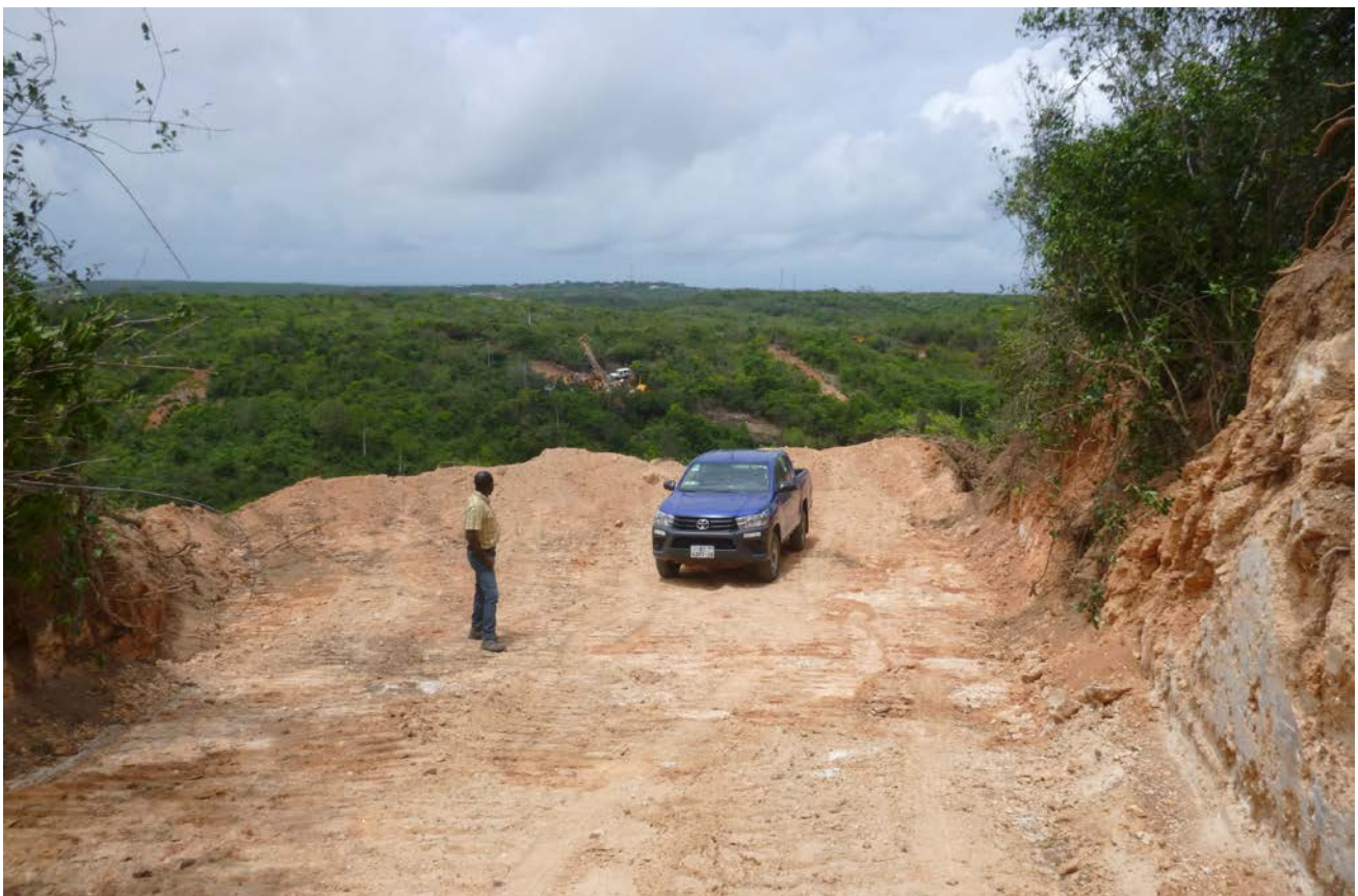
Figure 6 | View looking South towards drilling now underway at the Southern target zone.
