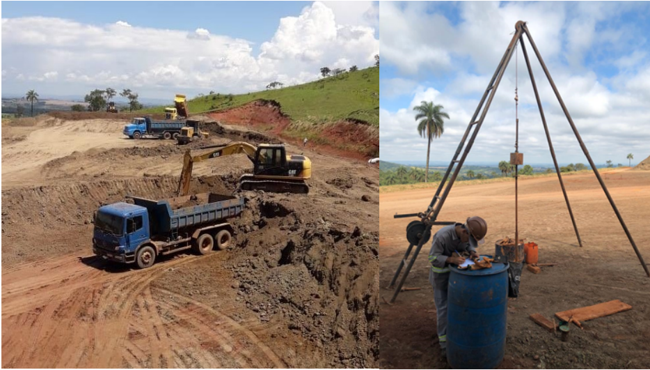
Figure 1: Initial groundworks underway for the product storage facility expansion
