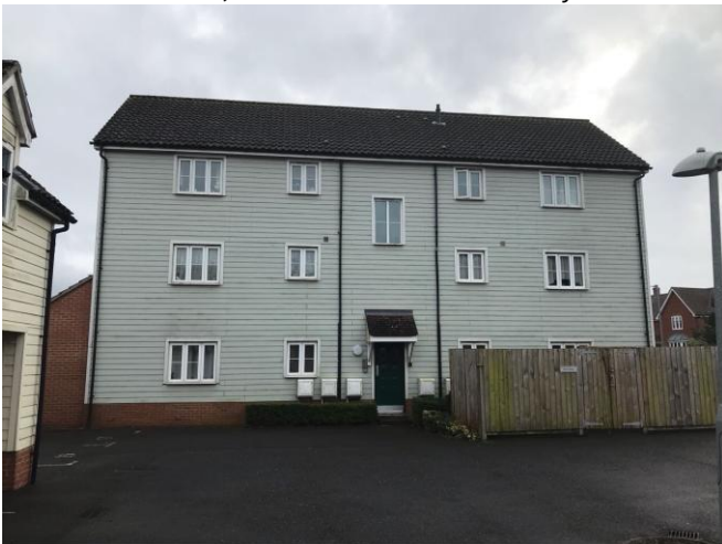
NR5 0UL, Bristol Road New Costessey - 1
