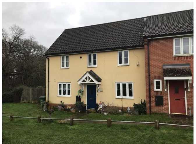
NR5 0UL, Bristol Road New Costessey
