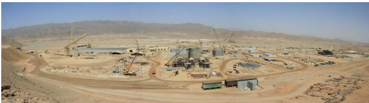
Progress Picture 2: Sukari Plant Site
