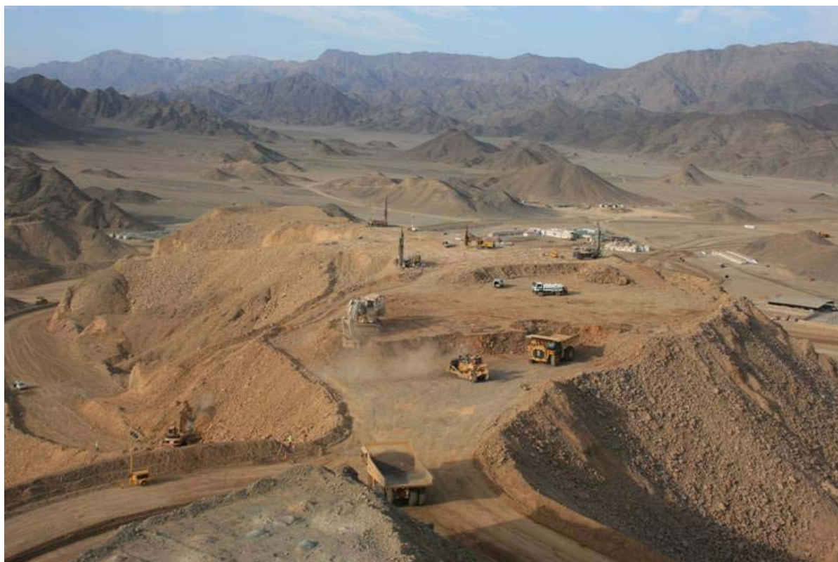
Progress Picture 3: View of current mining activity at Sukari
