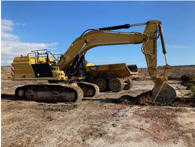
Figure 1: Breaking Ground for the installation of X-Ray Transmission (“XRT”) Ore Sorters
