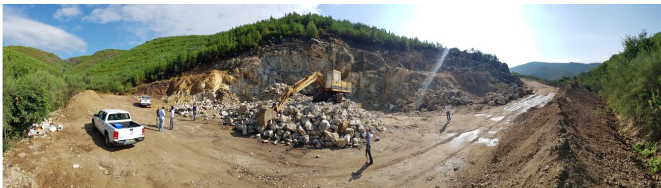
Figure 2. Panorama Photo of the Pegmatite Quarry on Block A
