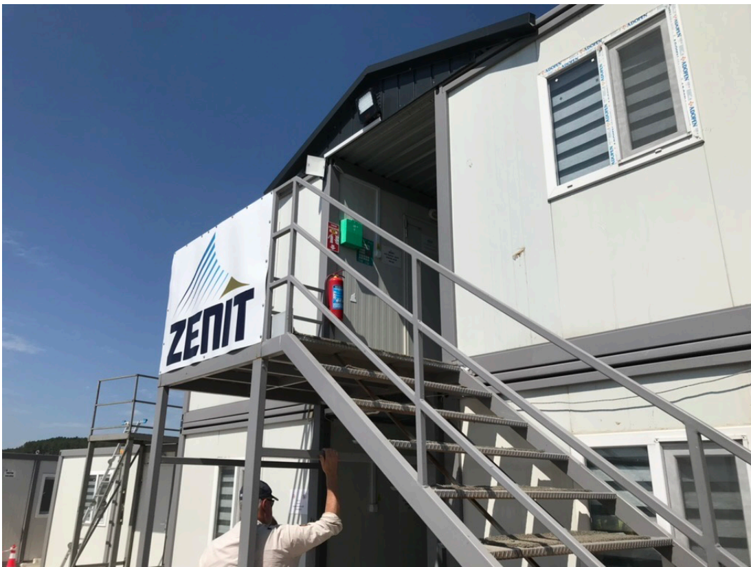
Figure 3: Construction management office at the Tavsan Mine site.
