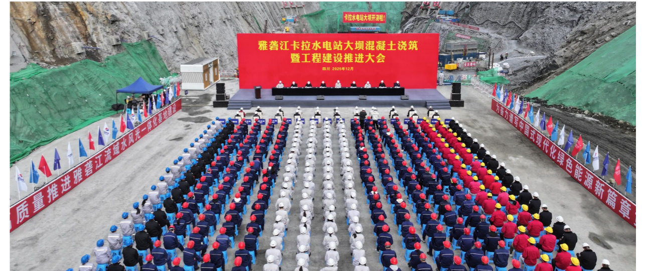
Concrete pouring for the dam at the Kala Hydropower Station of Yalong Hydro has begun.
