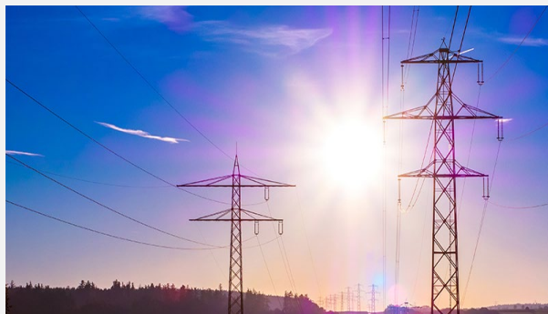
The project's 12MW power demand will be sourced from existing national grid supply lines. Alternative power sources may be accessible in the future when various renewable energy projects become operational.
