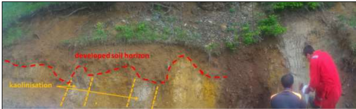
Figure 10 – An exposure located at Khatinca, showing strong oxidation of the weathered zone (with patches of kaolin-rich alteration), capped by a soil horizon.
