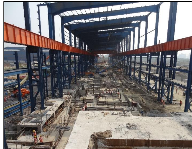
Entry side equipment foundation of PLTCM
