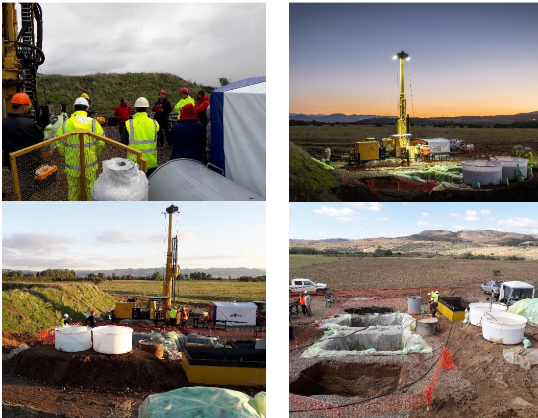
Figure 1: Site Preparation, Safety Briefing and Drilling: KMSL-4
