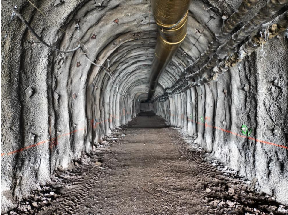
Figure 2: Underground at the Upper Portal
