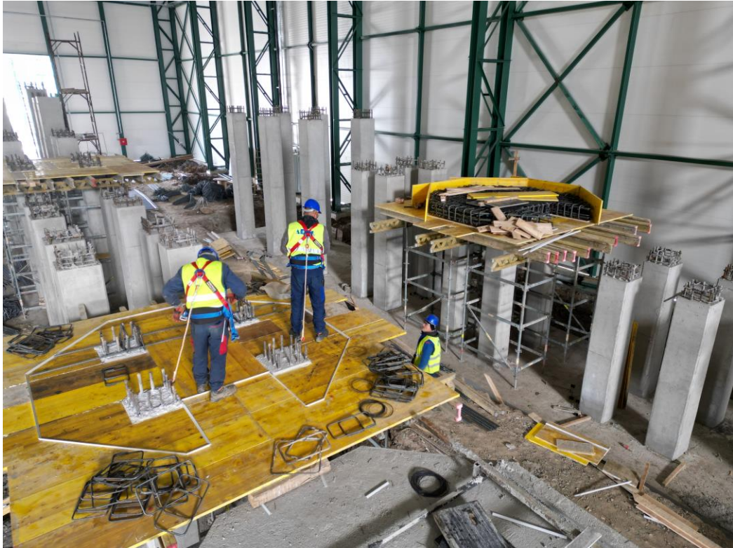
Figure 6: Inside the Vares Processing Plant
