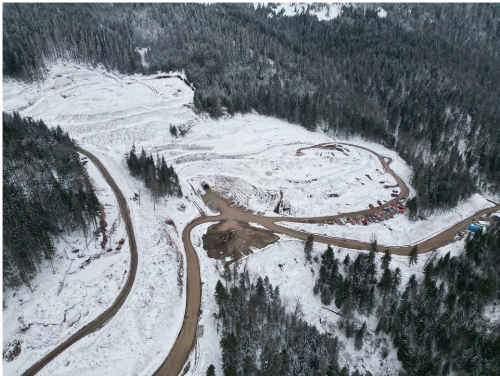
Figure 3: Upper Decline Portal
