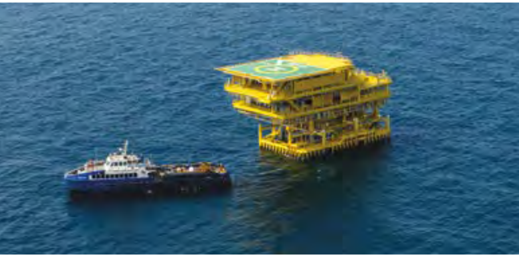
▲ Newly-installed wellhead platform Arabian Gulf
