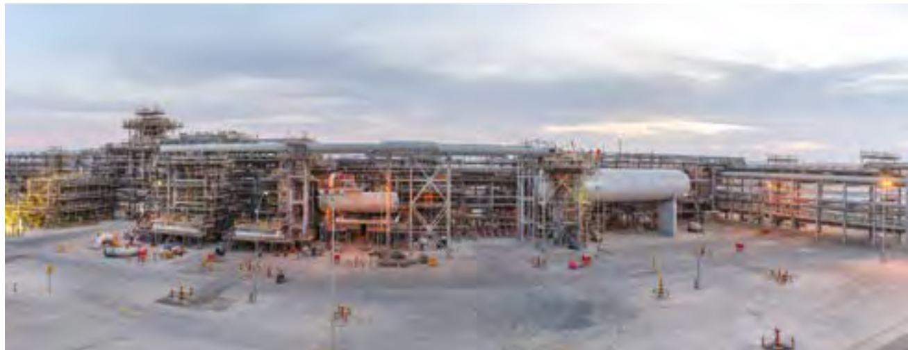
▲ Hawiyah Gas Plant Saudi Arabia
