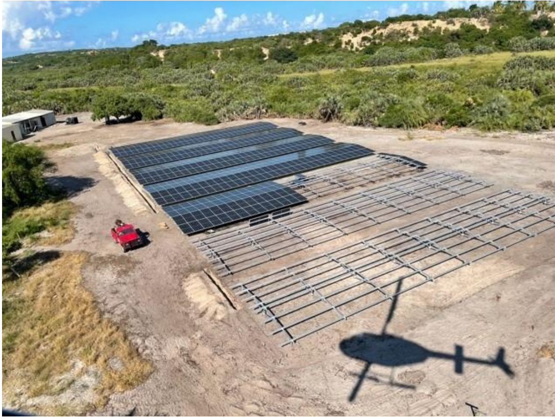
Image 1: Solar panels going up on site
