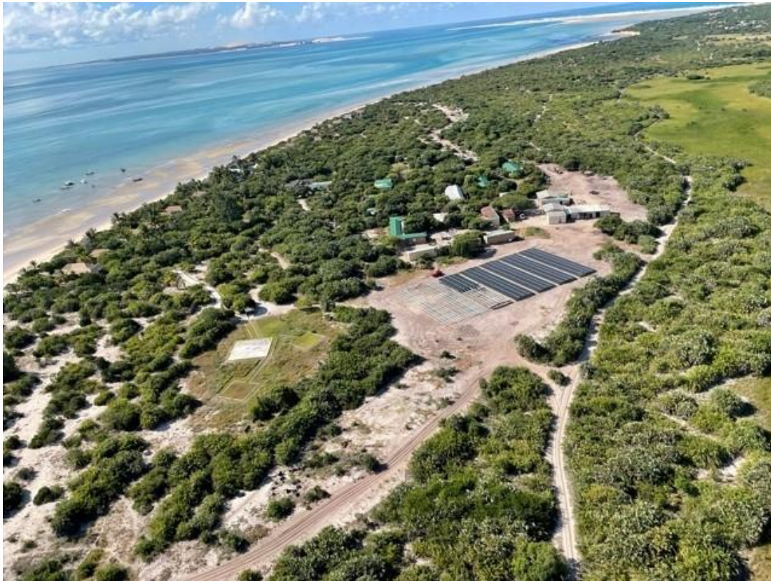
Image 2: Aerial view of solar panel installation and site clearance
