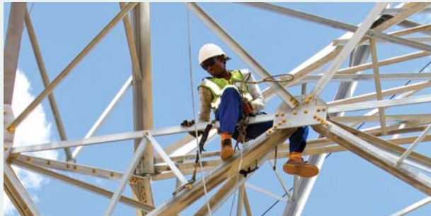
Working on transmission lines for Eskom
