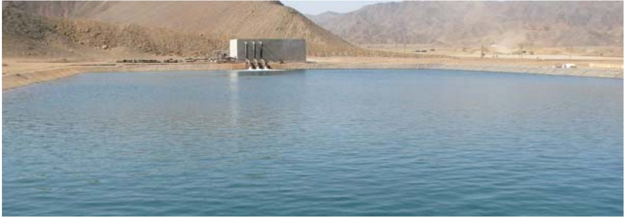
Above: Raw Water Pond at Sukari filled to capacity following successful intake from the 25km pipeline
