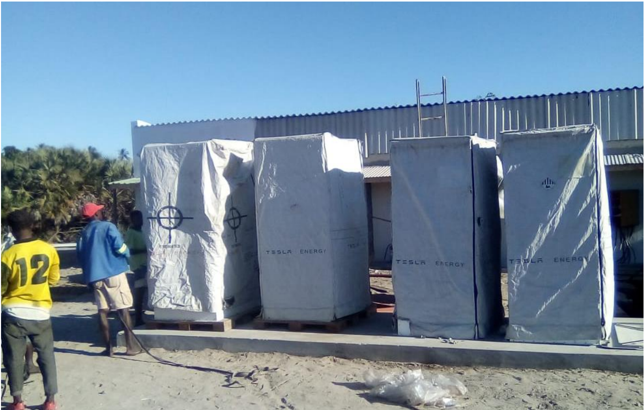
Image 1: Tesla Power Pack's being delivered on site
