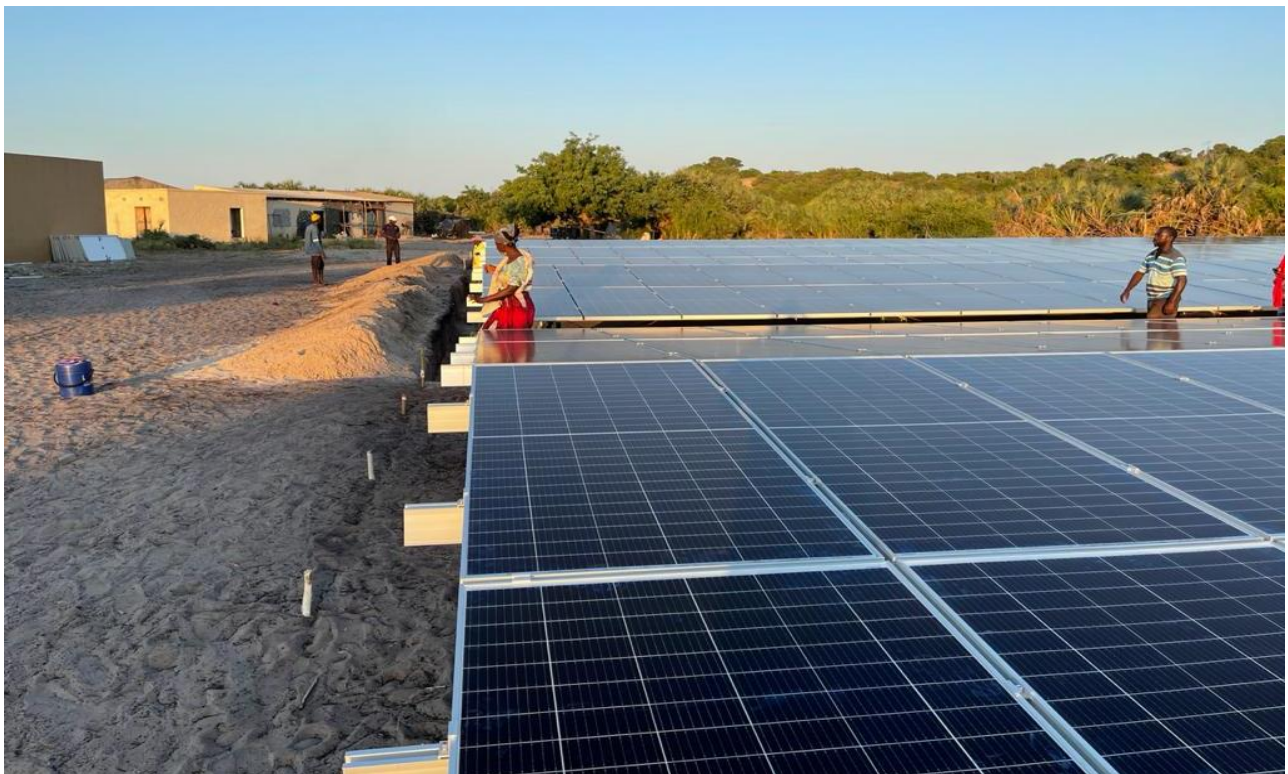
Image 2: Solar PV panels fully installed
