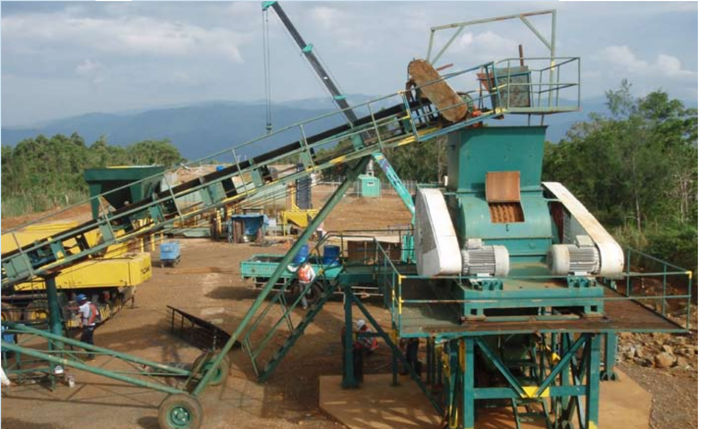
Rolls crusher under commission
