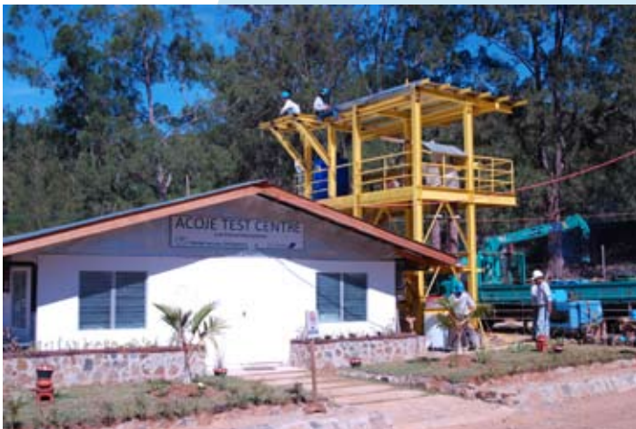
Acoje Test Center. 4m test columns being installed at rear
