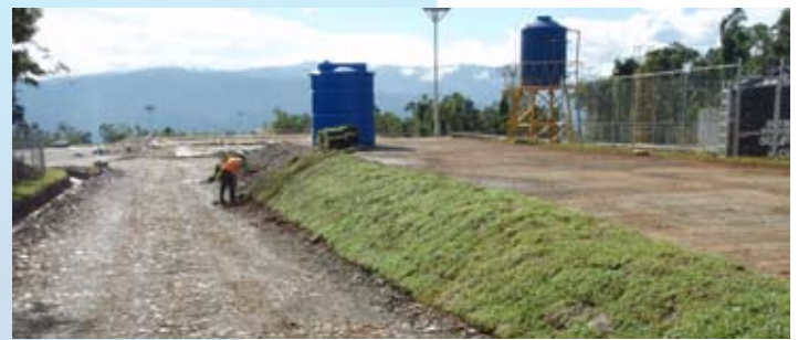
Landscaping at loading ramp
