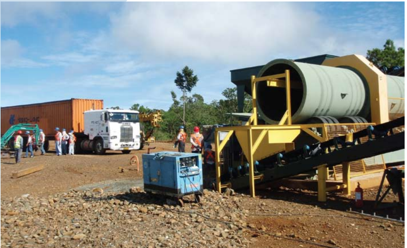
Crusher arriving on site with agglomerator in foreground
