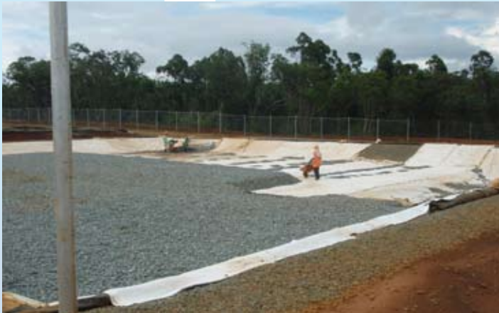
Acid resistant pebbles being laid in pad
