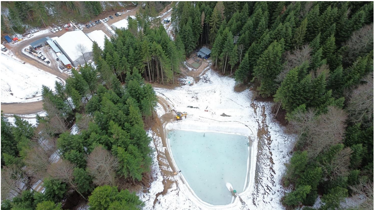
Figure 7: Water Treatment Plant, December 2023
