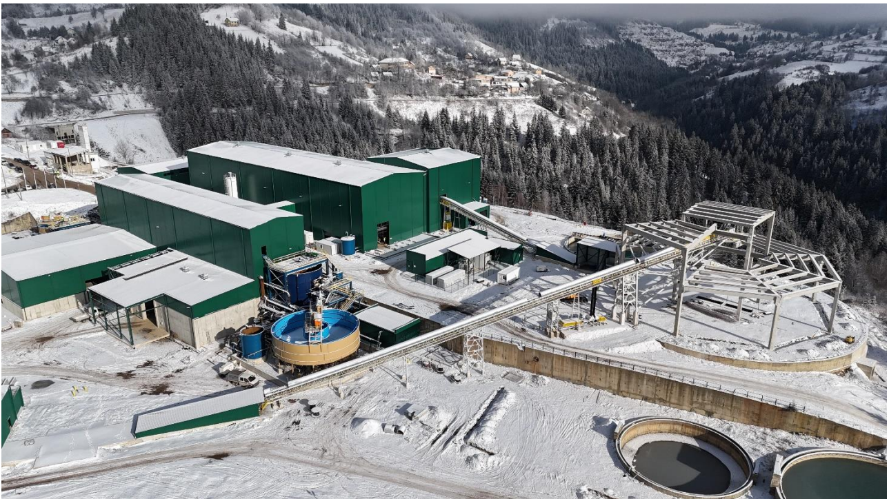
Figure 13: Aerial view of the Vares Processing Plant, January 2024
