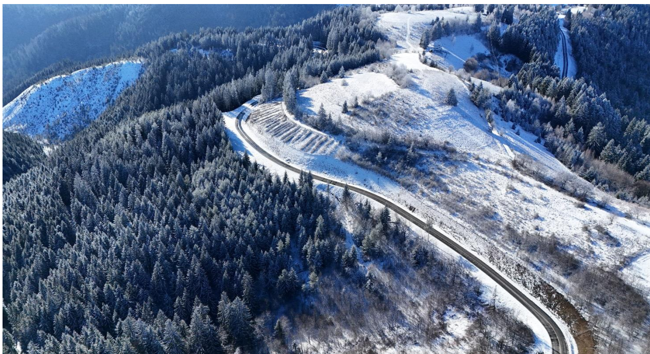
Figure 14: Aerial view of the completed road, December 2023
