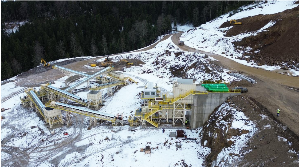
Figure 8: Crusher Plant, December 2023
