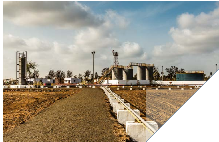
Figure 5: Bhandut Production Facility
