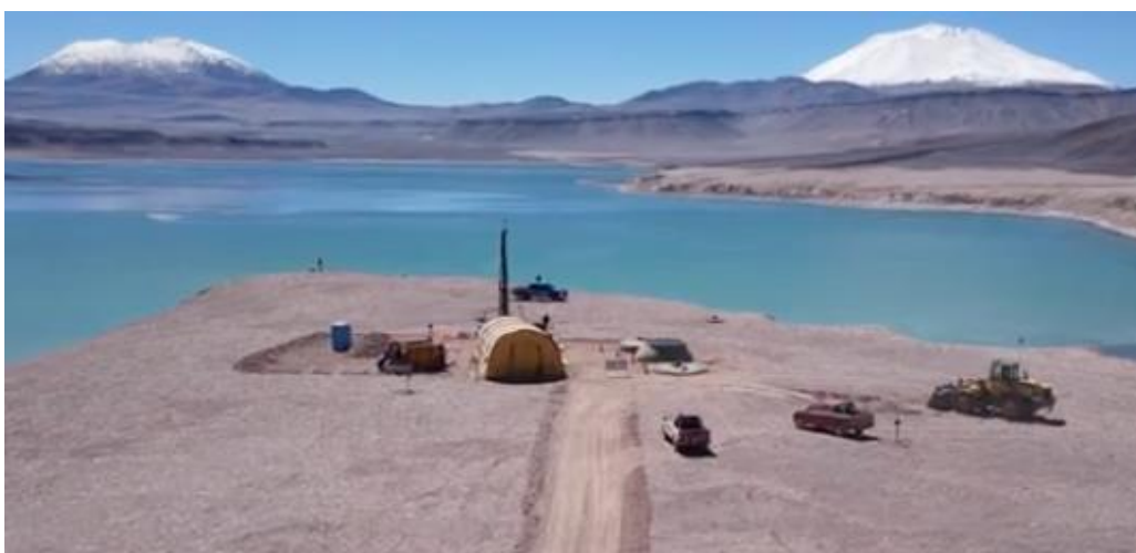
Fig. 6: Drill Rig and Auxiliary Equipment at LV01, 1Q 2022
