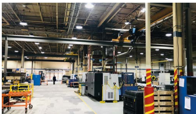
LED Lighting Installation in Canada
