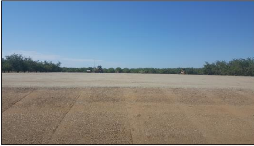
Completed Drill Pad
