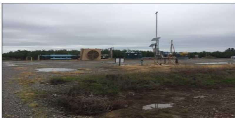
Dempsey Drill Site prior to construction
