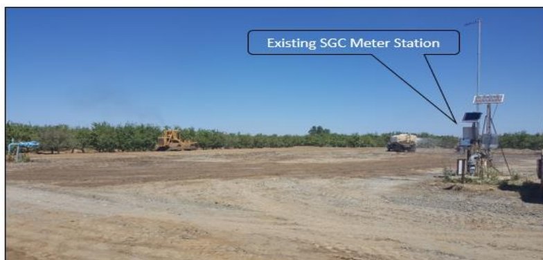
Driling Pad under construction
