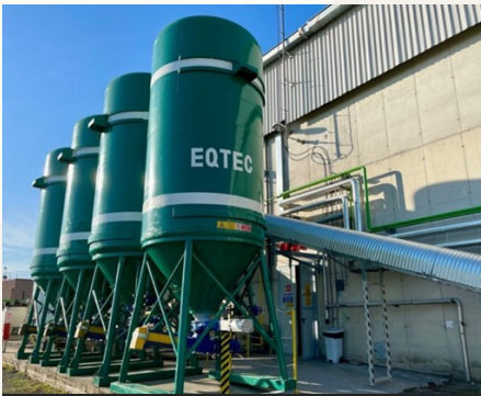
Four external hoppers capture approximately five days' worth of biochar output by the thermal cracking reactor inside the plant.
