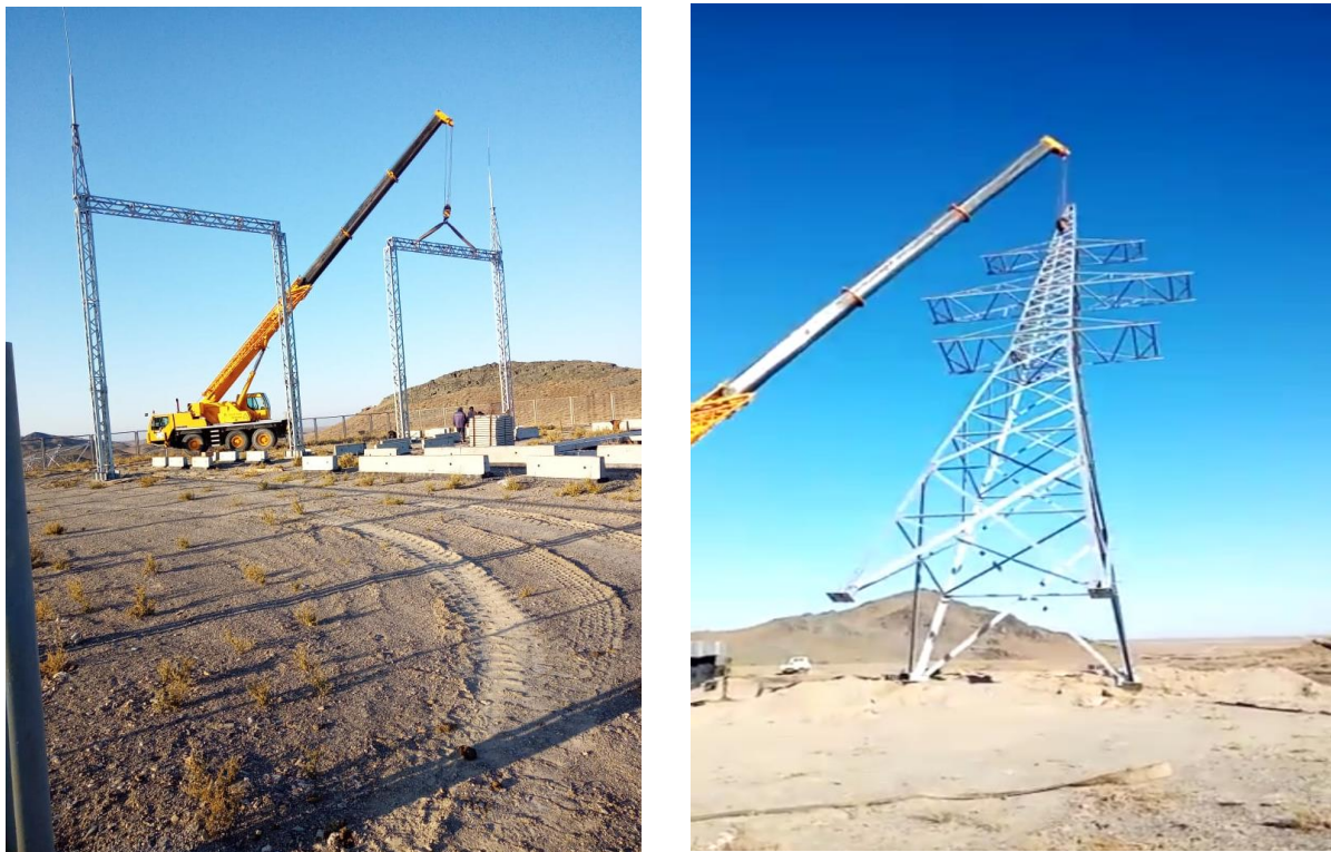
Figure 1: Work on the construction of the high voltage power line
