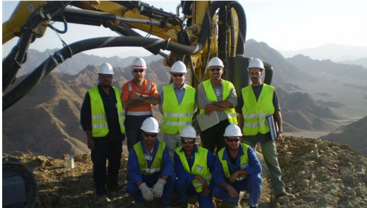
Progress Picture: Blasting Crew on the Sukari Hill
