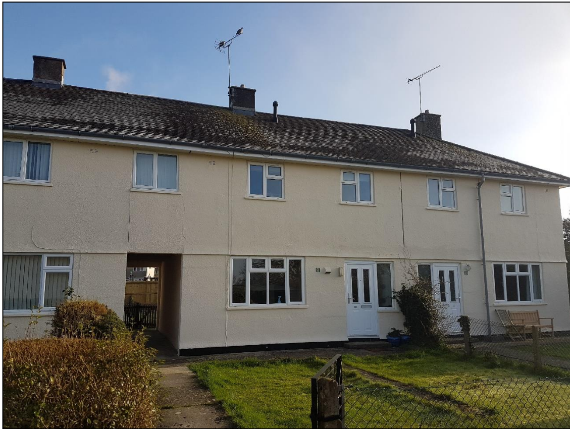
51-53 Paterson Road, Cirencester, Gloucestershire, GL7
