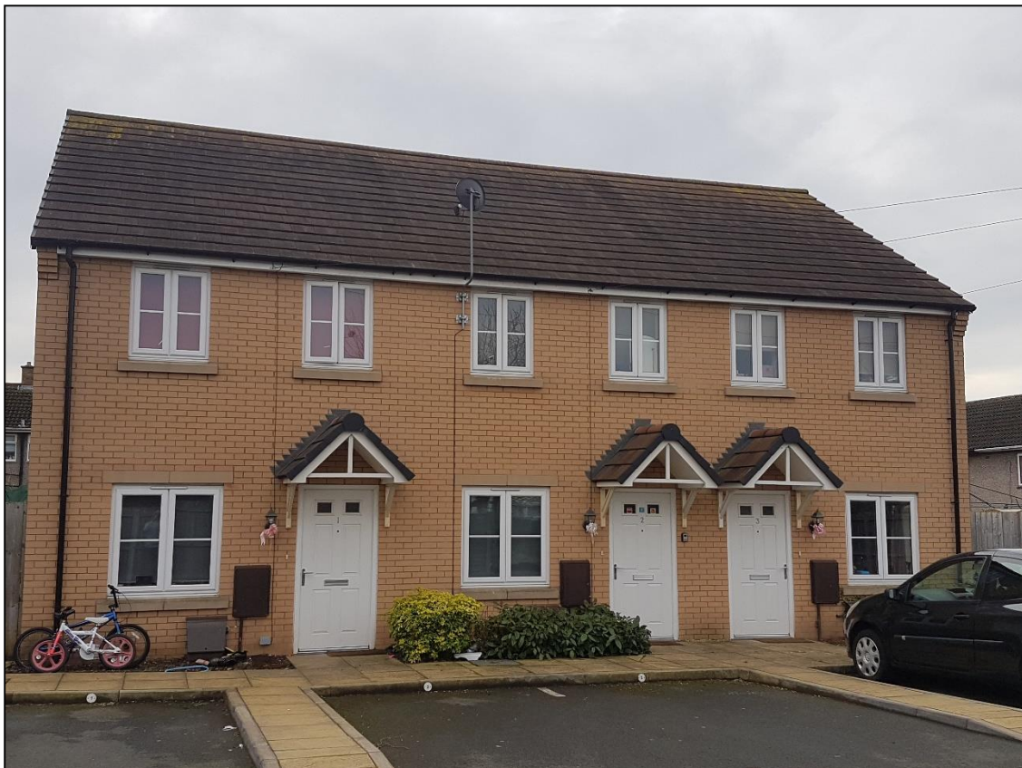
1-3 Marlowe Court, Mansfield Drive, Tamworth, B79
