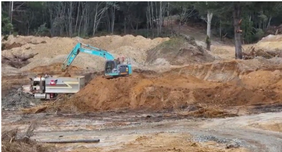
Figure 2: Excavation in the Wetlands environmental cleanup area.
