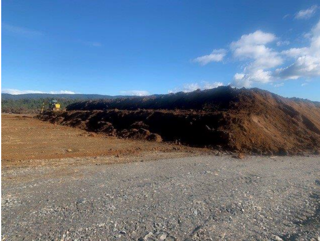
Figure 1: Beaconsfield Wetlands area deposited near the Processing Plant.
