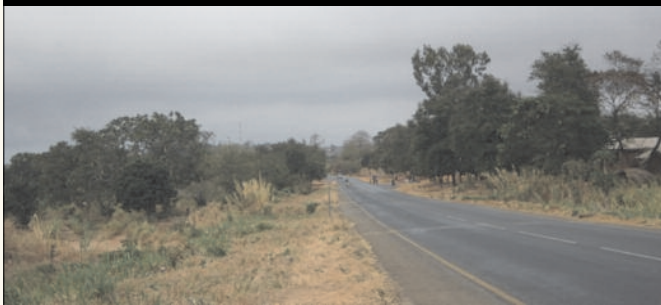
TAR ROAD TO DODOMA BLOCK AREA
