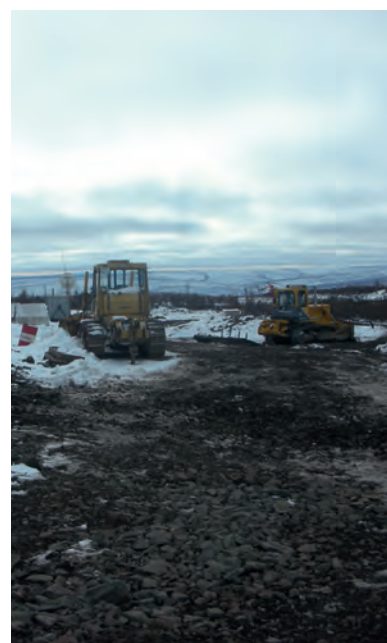
Bulldozers at Podgorniy camp
