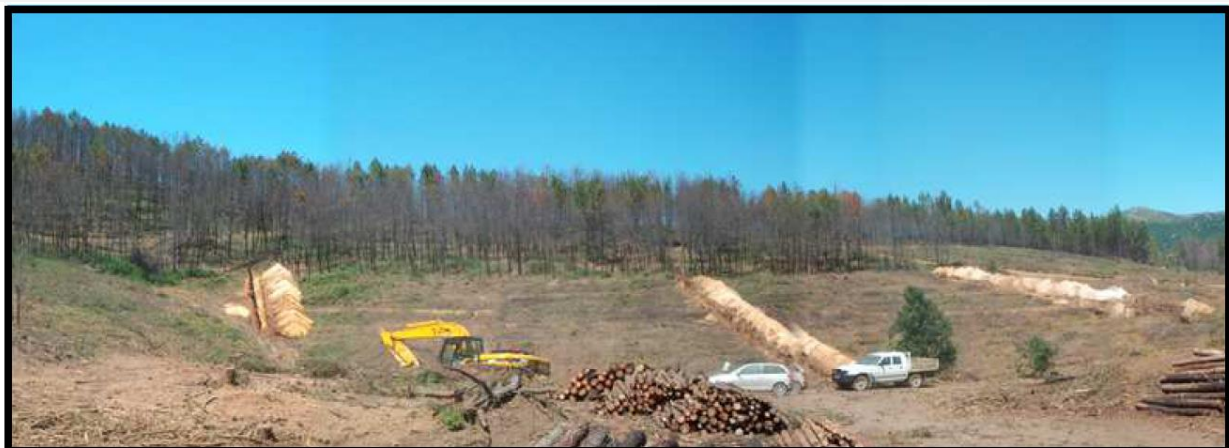
Figure 8. 2002 trenching being conducted
